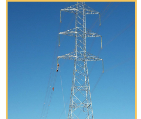
Sigdo Kopper LAT 500/220kV Mejillones - Cardones 900km line four bundle hardware & fittings and spacer dampers.
