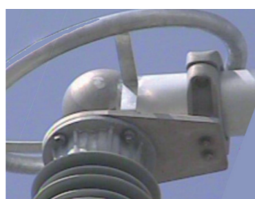
No corona detected, as expected from corona simulation.
